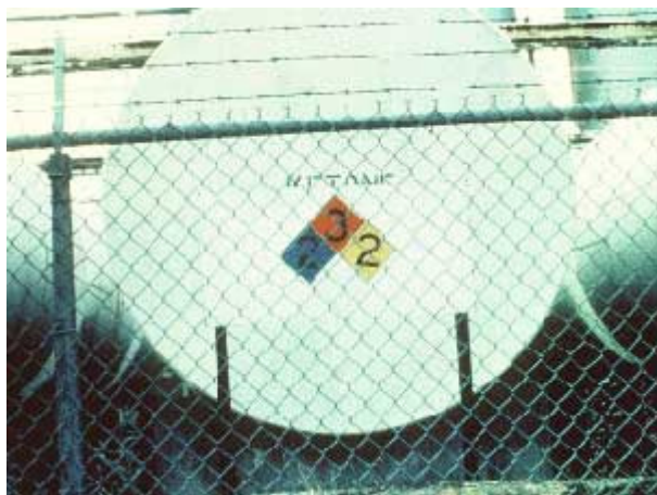
Figure 2-1, Example of NFPA 704 System
